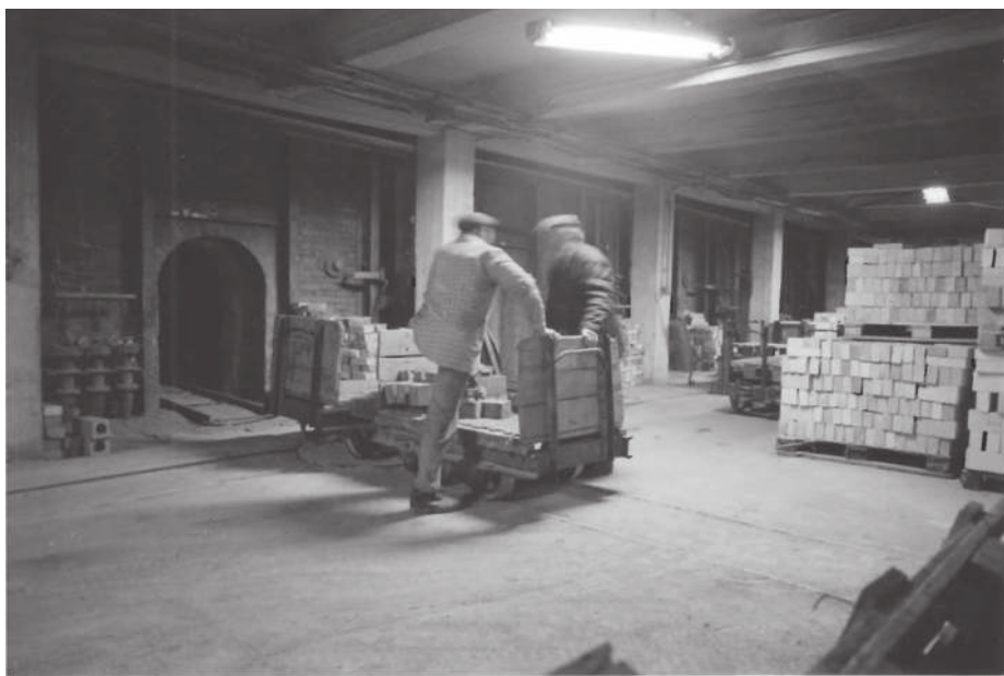
These brick-drying kilns provided the best protection from the icy winds.
